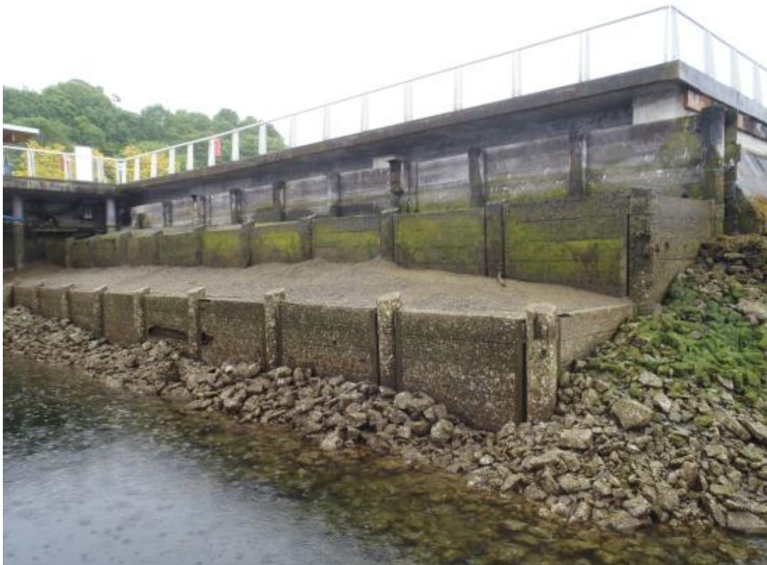
Seawall Overview (at zero tide)
